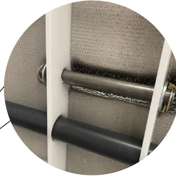
*Our pools are equipped with special supporting ribs that serve to stacking - ribs other than those designated cannot be used for stacking. These ribs are always equipped with a so-called lifting tube with safety latches*
