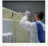
3. Application of an anti-corrosion fibreglass cloth
