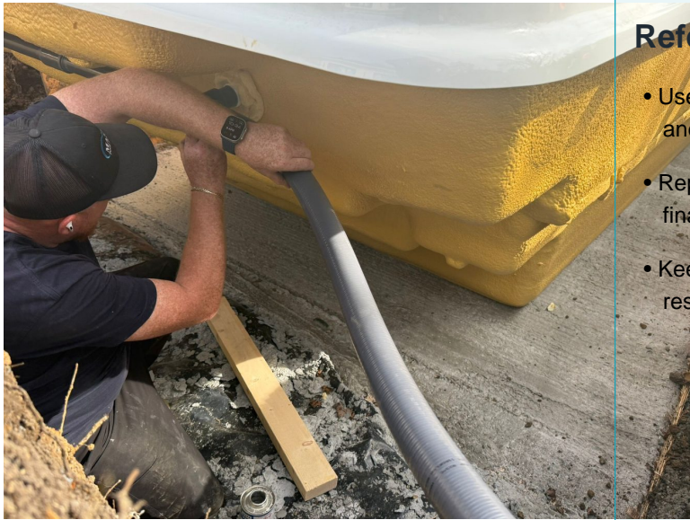
Reference photo: pipe routing and early connection planning.
