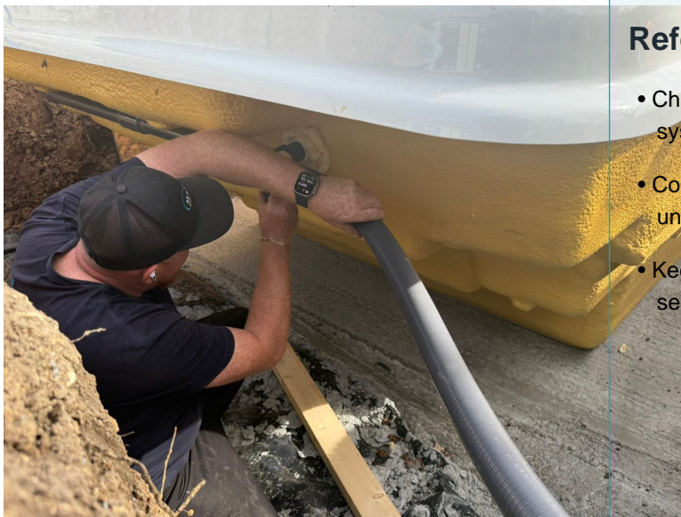
Reference photo: final pipework checking stage.
