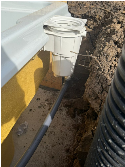
Reference photo: skimmer body and pipe connection area.
