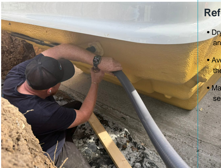
Reference photo: skimmer/pipe position for planning the route.
